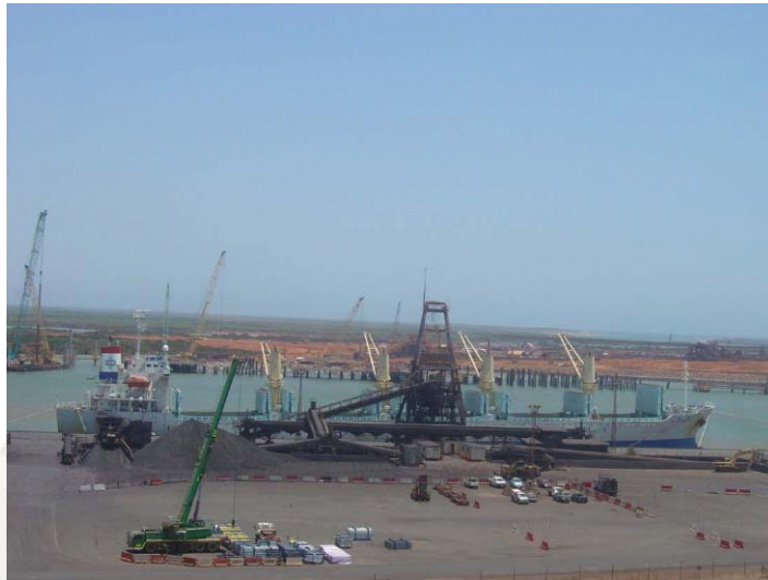
Inaugural shipment of Ant Hill ore being loaded at Port Hedland with new Utah Point berth construction visible across the harbour
